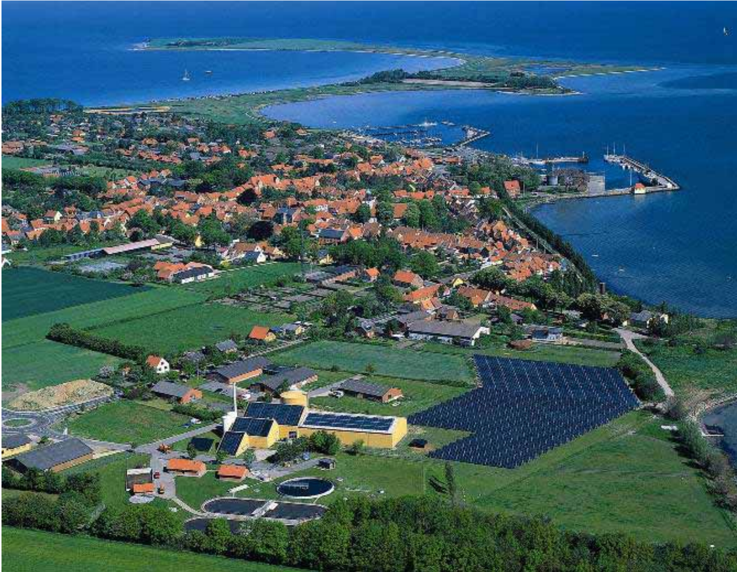
Solar heating and biomass plant, 4900 m 2 , Aeroesjøbing, Denmark Source: ARCON / ESTIF
