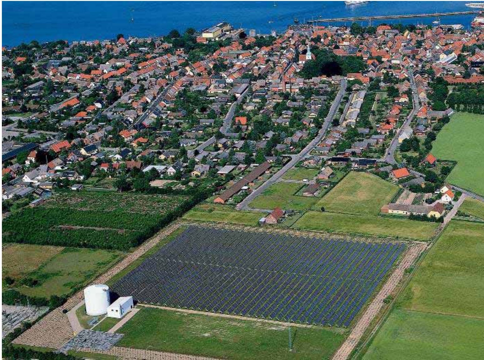
Europe's largest district heating solar plant, 20000 m 2 , Marstal, Denmark Source: ARCON / ESTIF
